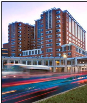
New pavilion A at UK Albert B. Chandler Hospital
