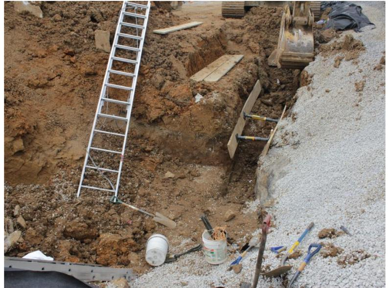
**Figure 2.** View looking down at the trench containing a mixture of class B and C soils on the right side of the trench near the concrete wall. Class B soil is observed on the opposite side of the trench.
