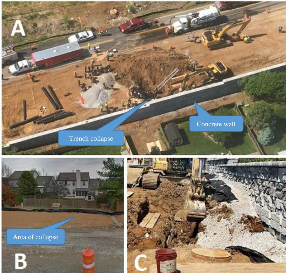
**Figure 1.** A) Aerial view of incident scene, B) photo of trench collapse location 4 months prior to incident, C) section of trench that collapsed on victim; concrete wall.
